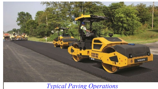
Typical Paving Operations
